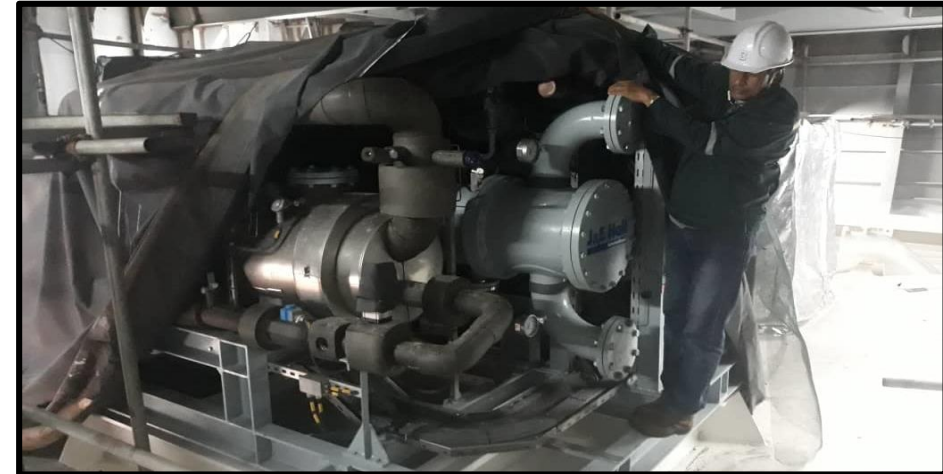
Chilled water plant installation
