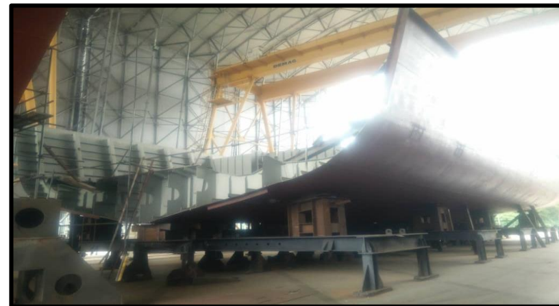
Main block erection
