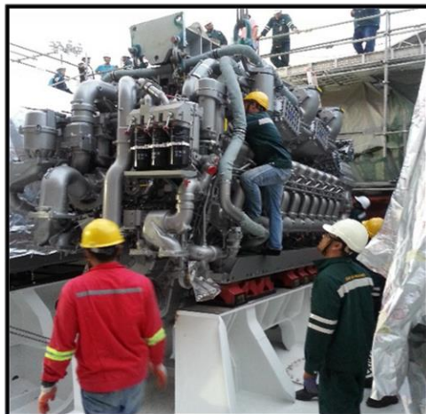
Main Engine Installation
