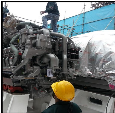
Main Engine Installation
