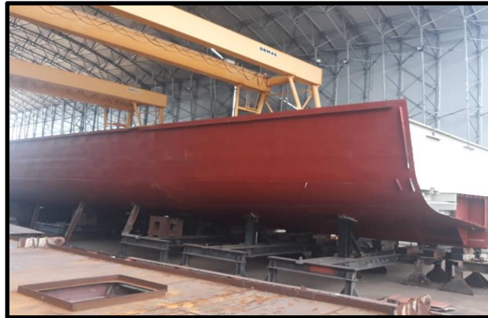
Main block erection
