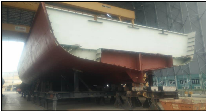
Main block erection
