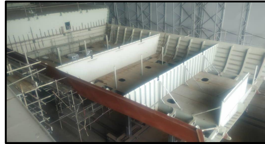
Main block erection
